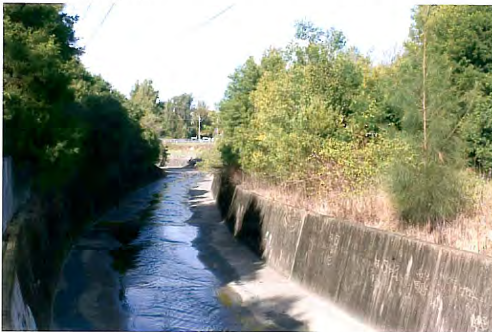
Figure 2 – Concrete Lined Cooks River
